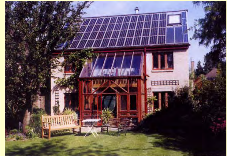
Figure 3.24 In this solar house in Oxford, UK, a 4 kWp grid-linked array of monocrystalline PV modules forms an integral part of the roof, alongside solar water heating panels. The PV array supplies the house's annual electricity requirements, plus a small surplus used to provide some of the power for a small electric car
