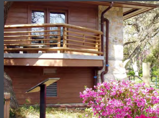
First-flush downspout device
