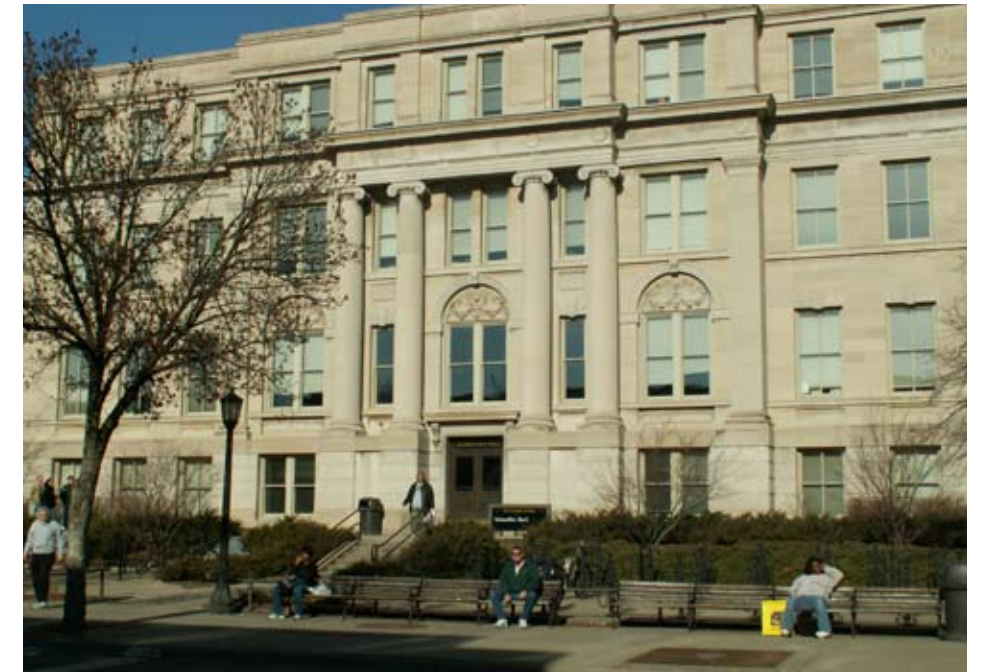
Today, there is a need to wisely plan for the renewal of existing facilities to meet the space needs of the future. Old Capitol and Schaeffer Hall (above) are the first two Pentacrest buildings to have received major renovations. Jessup, MacLean and MacBride will follow.
