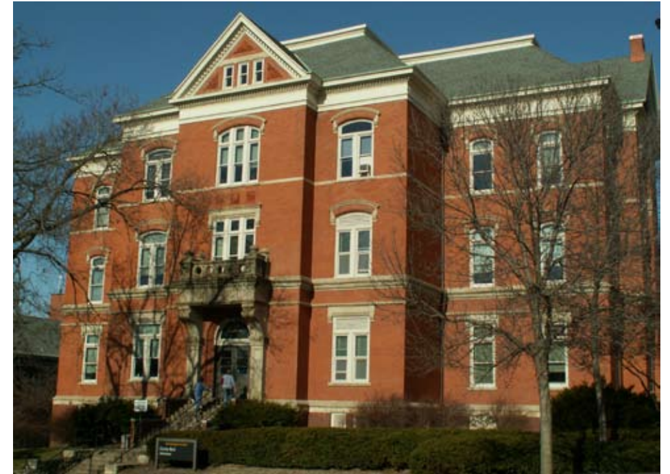
Renewal of existing facilities is recommended as a cost effective strategy to help meet the University's future space needs. Calvin Hall
