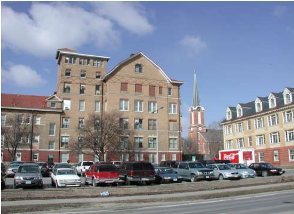
The planned renewal of Seashore Hall and Old Music will revitalize the east edge of the Iowa City Campus. This area contains buildings dating from 1899.
