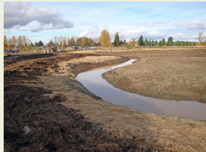
Treatment channel under construction
