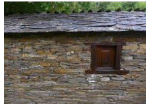
Techo de pizarra (slate roof)
